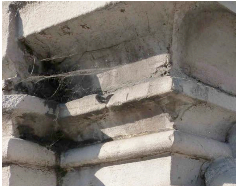
Fig 29: cornice made up with mortar on armature
