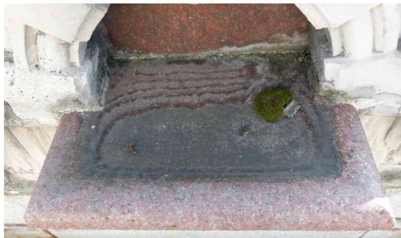
Fig 25: upper granite basin on west elevation
