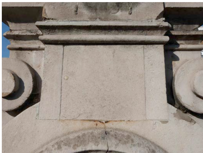
Fig 6: detail of east side showing removable panel
