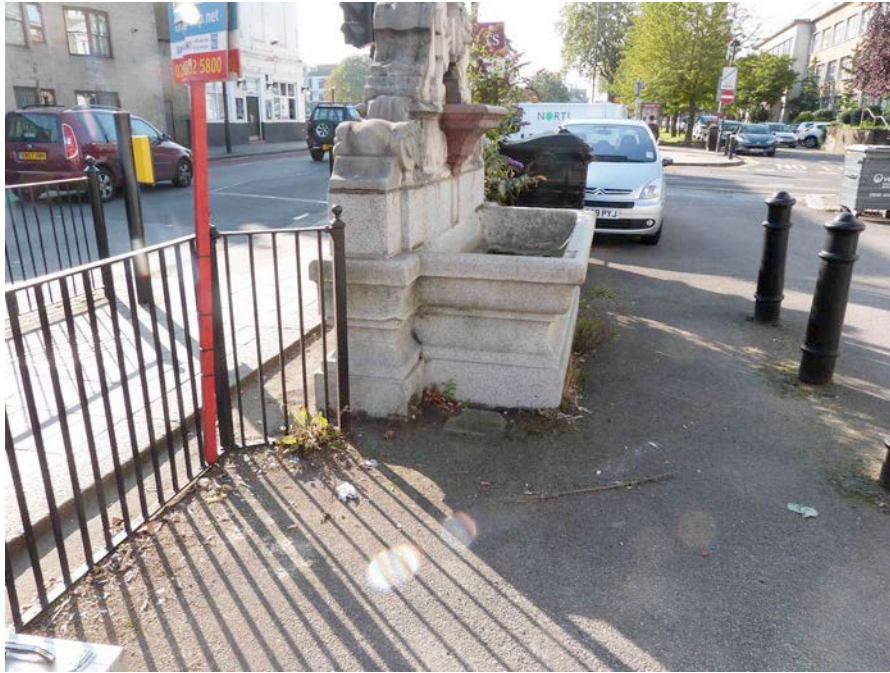
Fig 39: view of drinking fountain from north-west showing drain cover next to the trough
