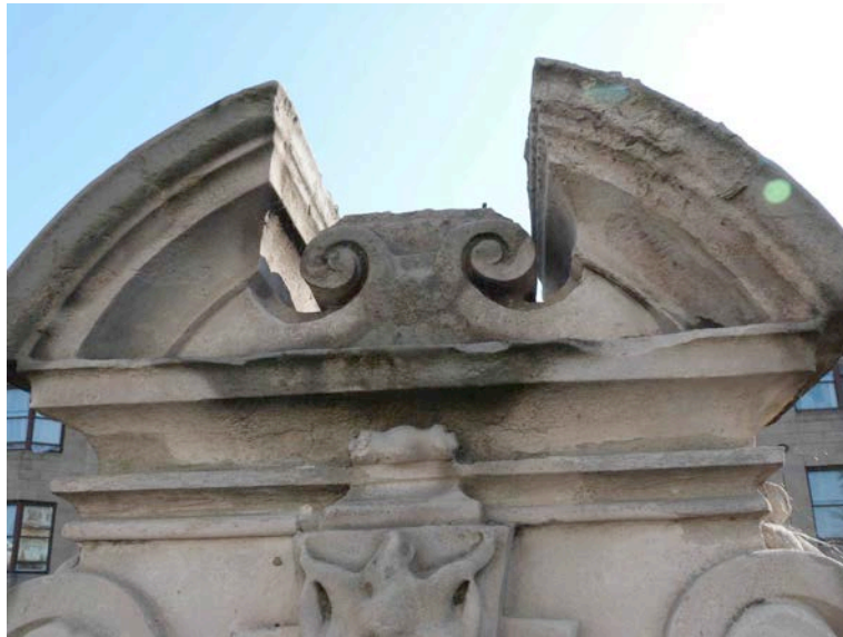
Fig 34: west side of pediment stone showing grey staining to stone
