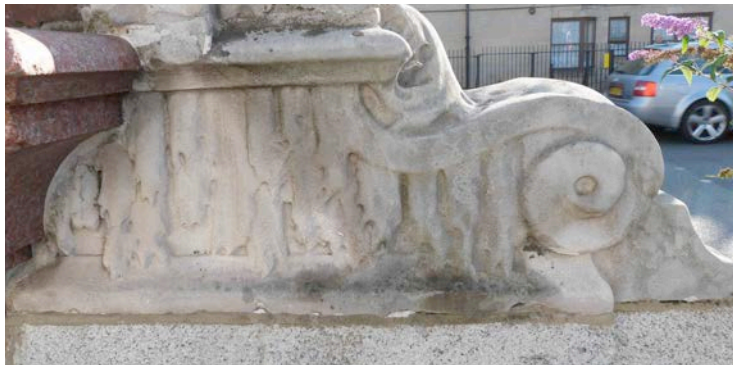
Fig 18: west side of south stone of course C
