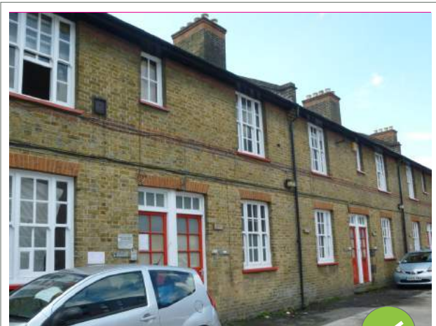
Original brickwork should be left exposed, and restored where necessary.
