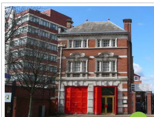
Change of use can result in the long term preservation of a listed building as in this example in the Tottenham Green Coconservation Area
