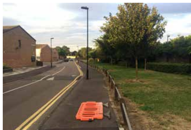
View eastwards along Fairbanks Road
