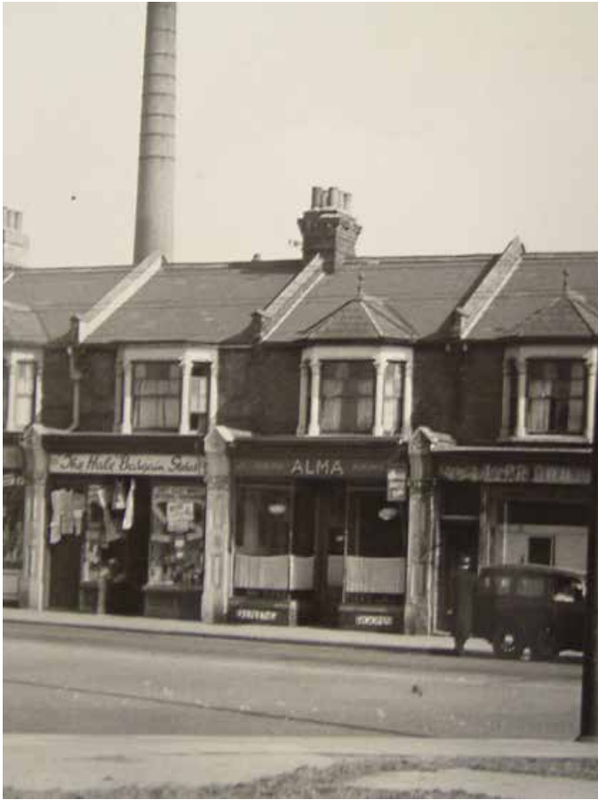
The Hale and factory chimney, 1955
