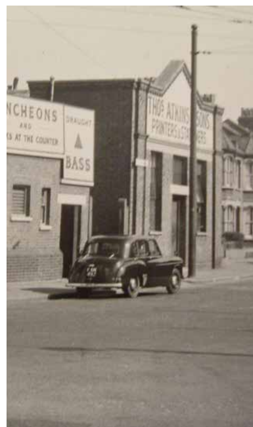
Station Road, looking west, 1955
