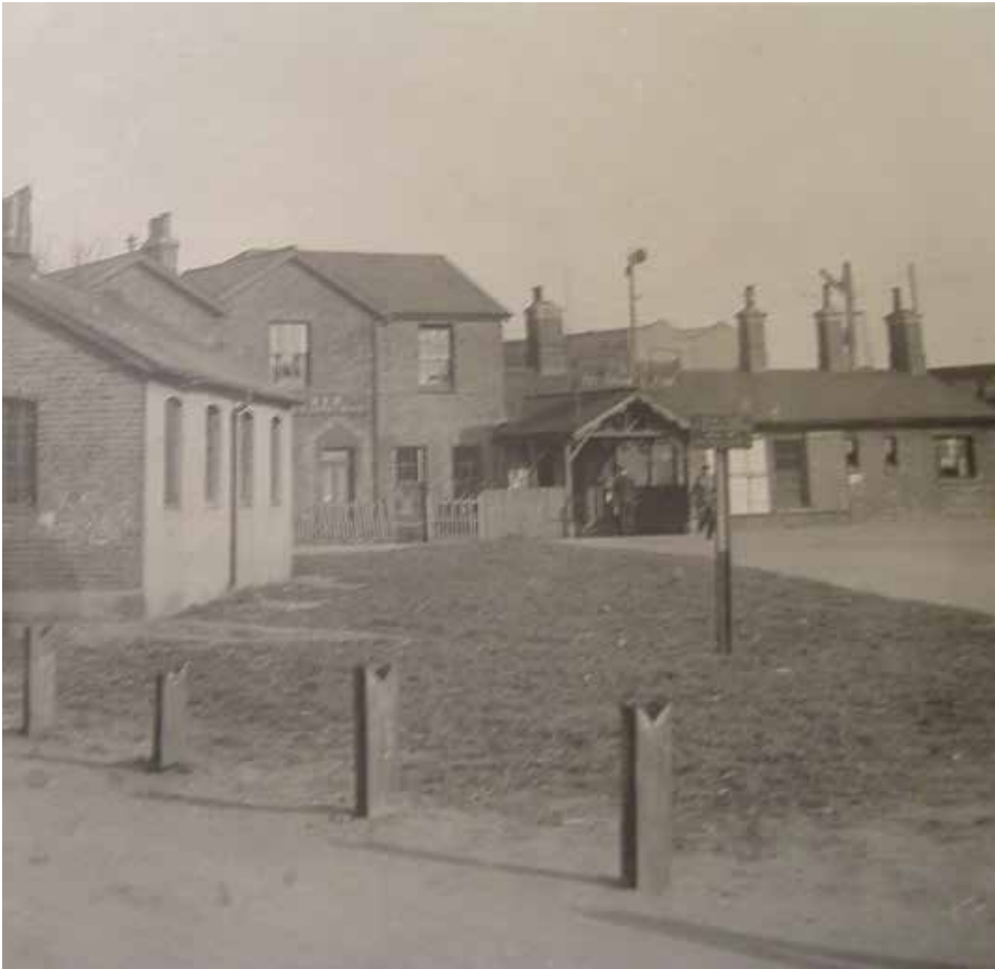
The Hale and factory chimney, 1955
