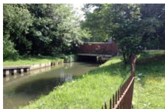
New River running under Station Road
