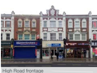
High Road frontage
