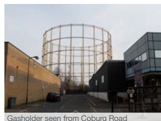
Gasholder seen from Coburg Road
