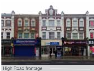
High Road frontage
