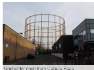
Gasholder seen from Coburg Road
