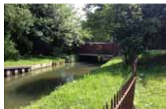
New River running under Station Road
