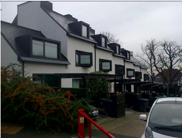
Recent development at 50-38 Connaught Gardens
