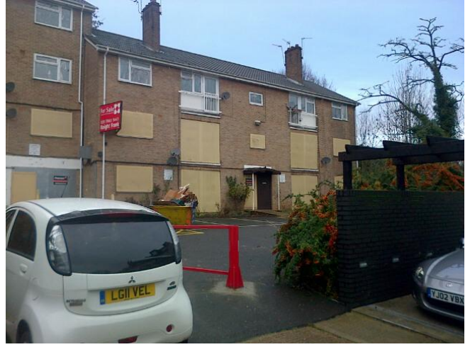
Existing front elevation looking north west
