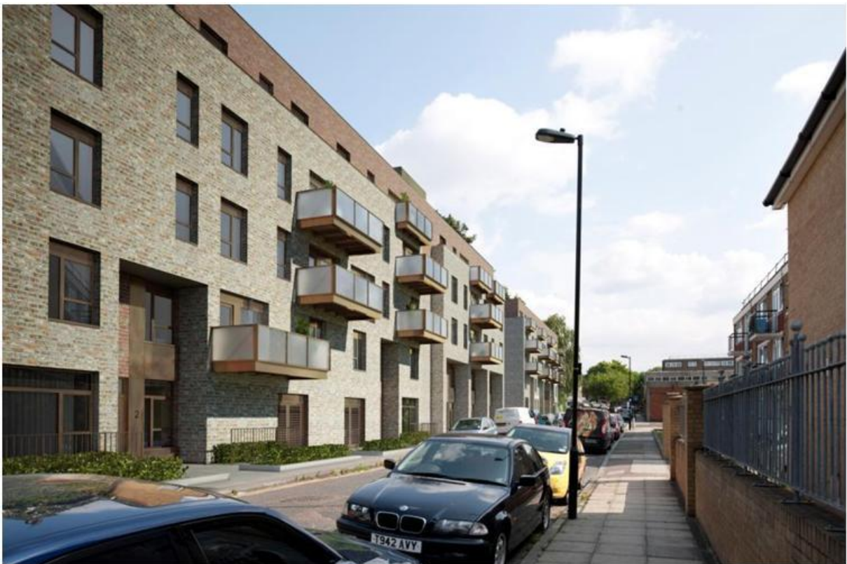
View looking south along Myddelton Road
