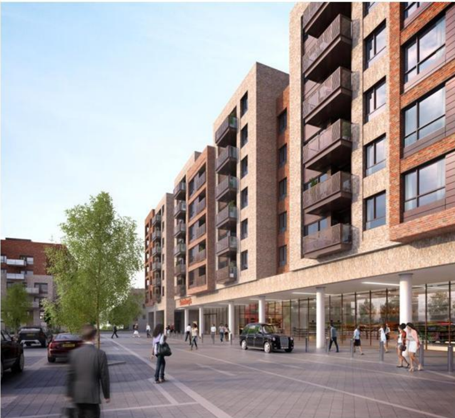
View from access road within site, just off High Street
