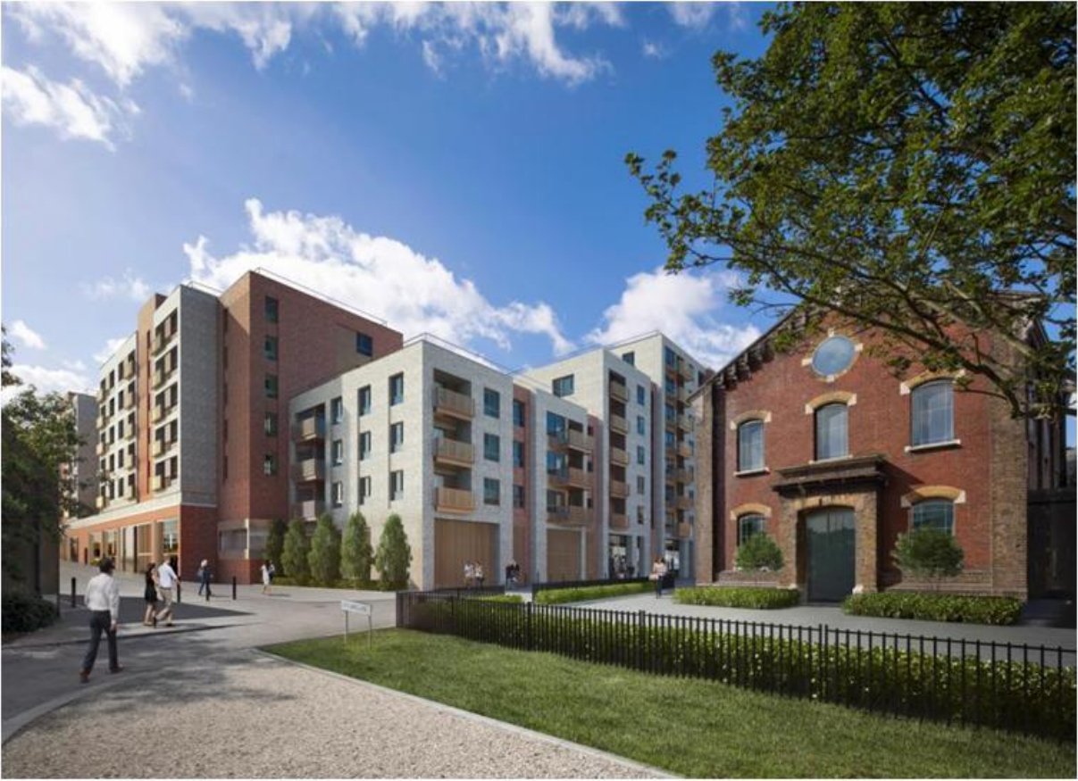
View from Great Amwell Lane looking south west
