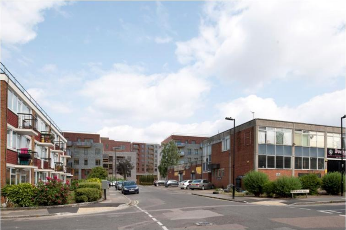
View looking east along Pembroke Road
