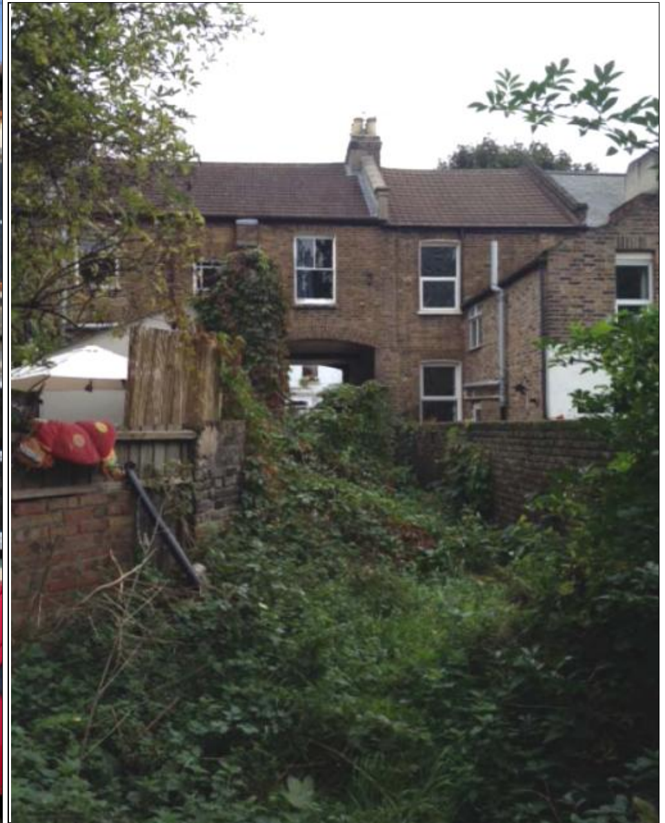
View towards access
