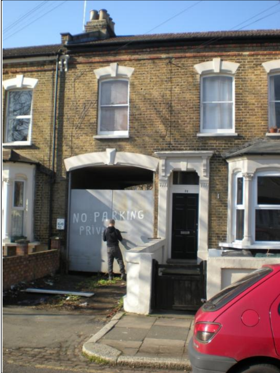
Existing site access on Beaconsfield Road
