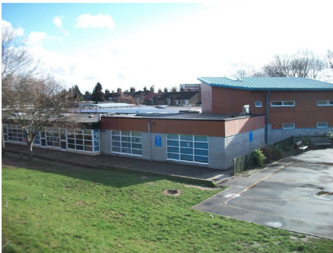
Existing School Building
