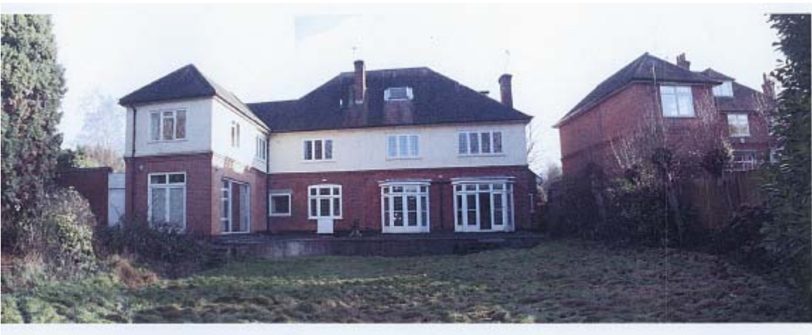
Western (Rear) Elevation
