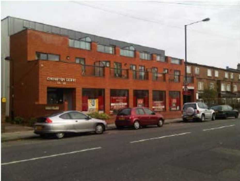
Photos 1 & 2 : Front elevation onto Mayes Road
