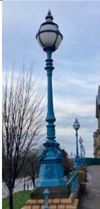
Figure 2, example South Terrace lighting column
