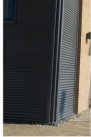
03 Cladding Profile - Sinusoidal
