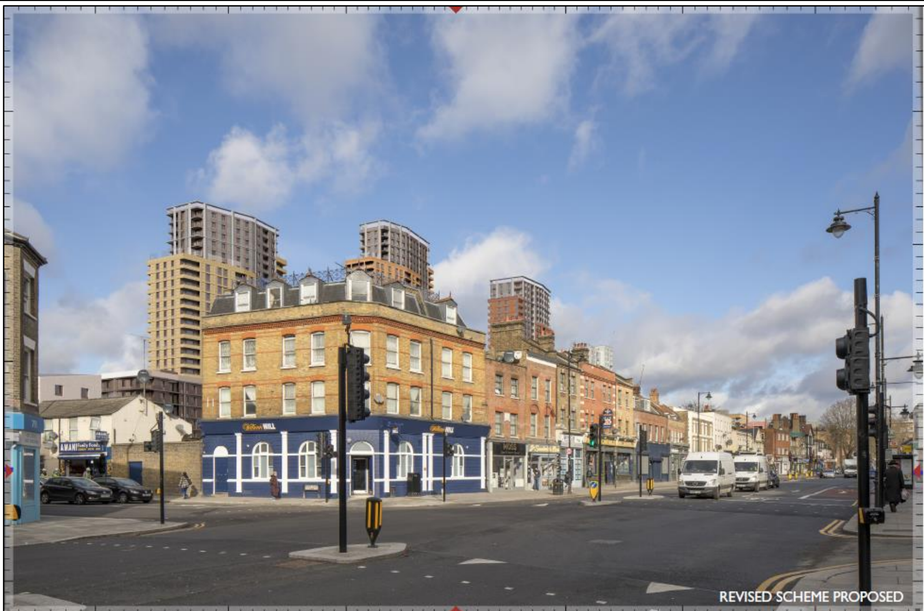
Looking north up High Road (next to Percy House) (View 5)
