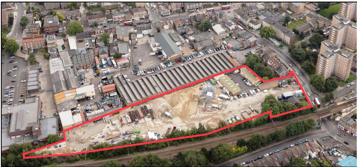
The Goods Yard site, looking east towards the High Road
