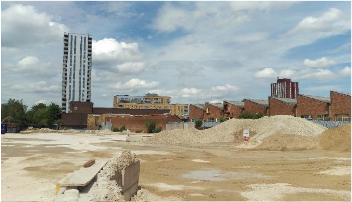
Image 1.4 – Existing Site Image looking northeast (Source Applicant)
