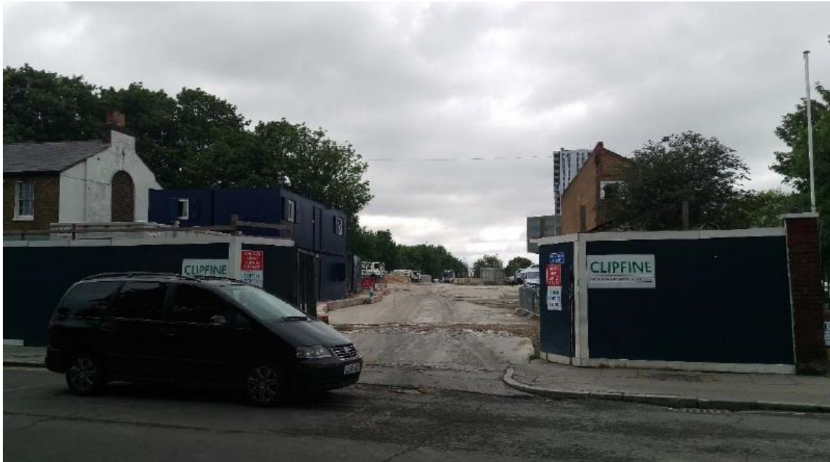
Image 1.2 – Existing Site access - looking north from White Hart Lane (Source Applicant)
