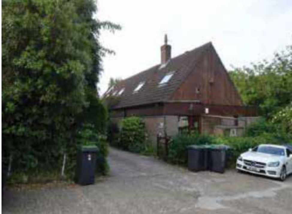
Site Photo – frontage of current building on site
