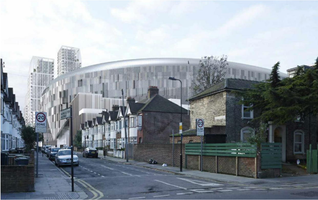
View of the Health Centre building from the end of Worcester Avenue
