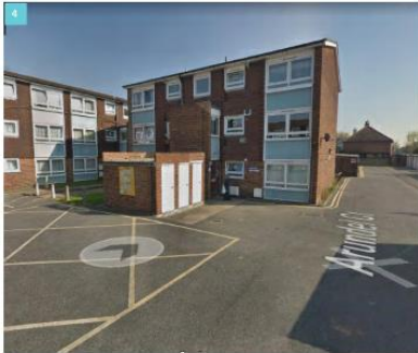
Parking area and the external pram sheds
