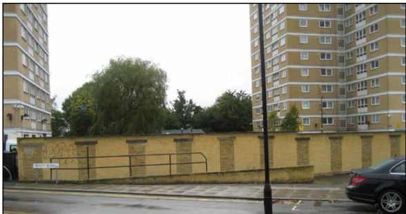
5.2 View of the bricked up garage doors along Trinity Road.
