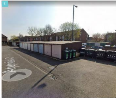
Garages and the external refuse arrangement
