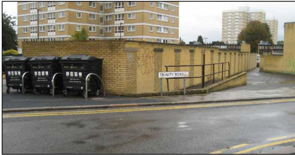
5.1 View of the bin storage area and the level change from Trinity Road to the rear of the site.
