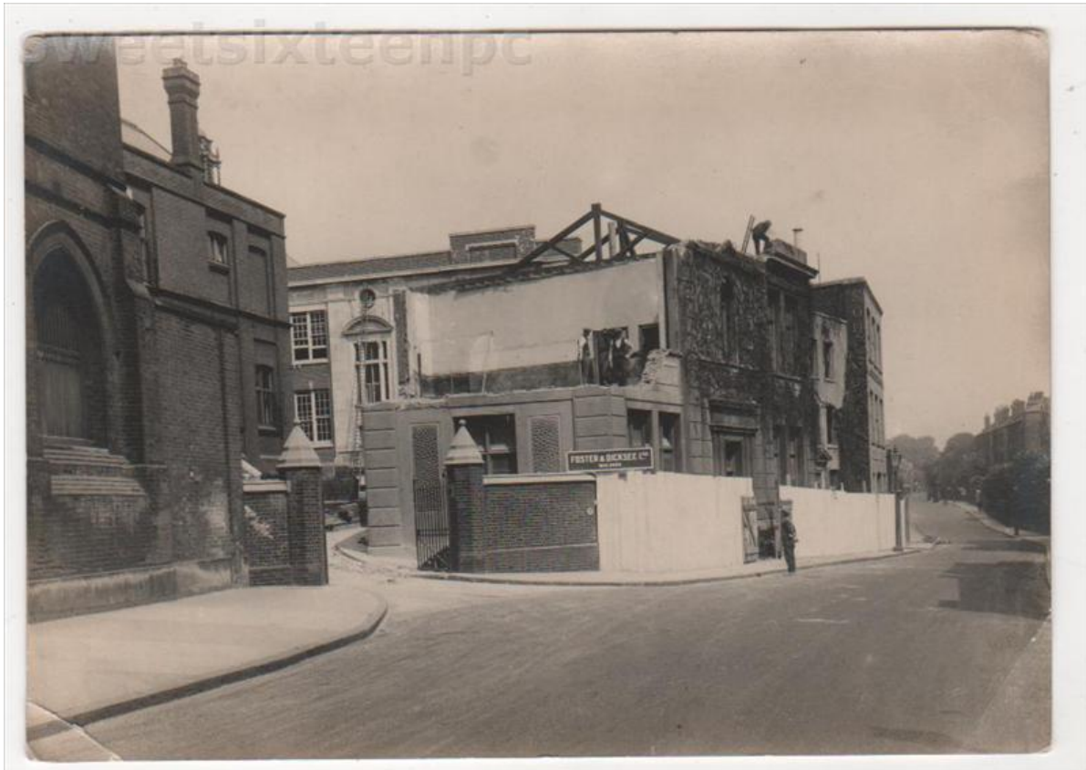
Photo 1: former British School (being demolished)
