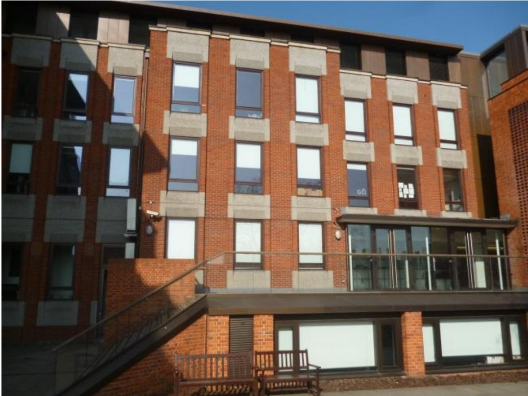
Photo 6: Garner Building (rear)
