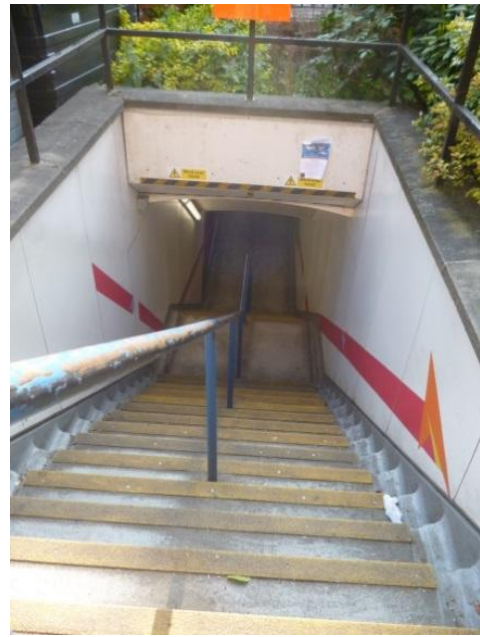
Photo 12: Southwood Lane Tunnel (entrance)
