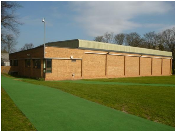
Photo 20: Sports Hall (Mallinson Sports Centre)
