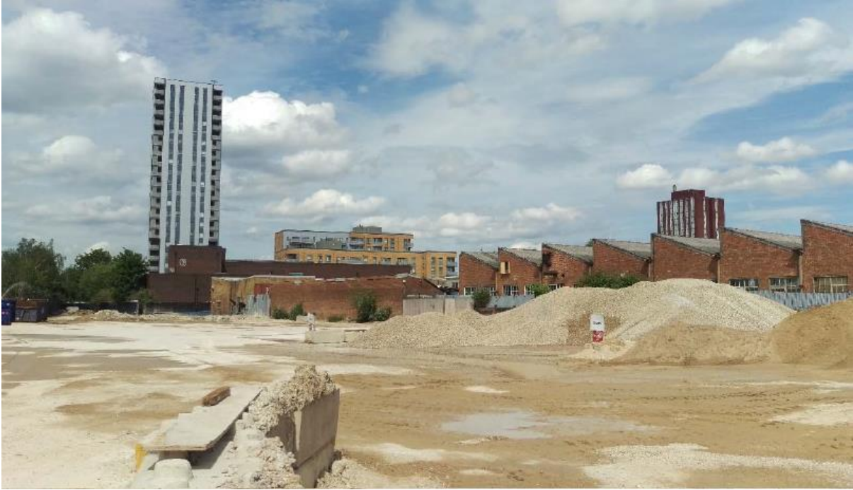
Image 1.4 – Existing Site Image looking northeast (Source Applicant)
