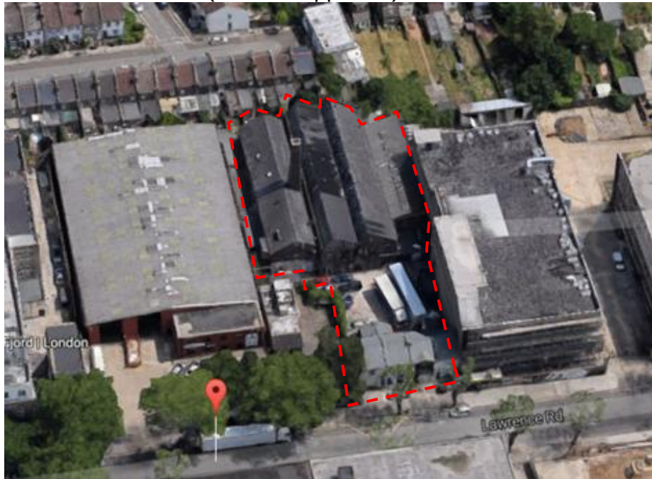
Image 1.1 – Historic Aerial Image - Looking East. (Source: Google Maps - Application site dashed in red for illustrative purposes)
