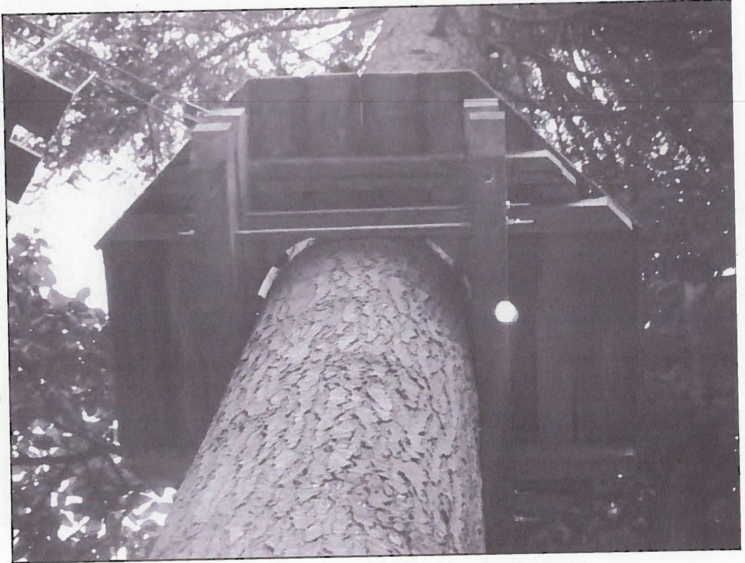
Example of Brace and Platform Construction
