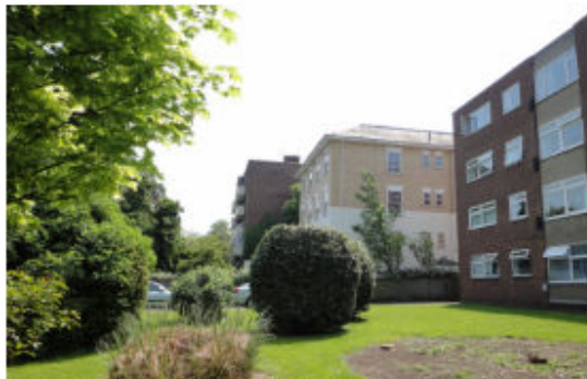
[05] photograph from Embassy Court's communal gardens and parking court with the application property and Rounde Green Court in the background
