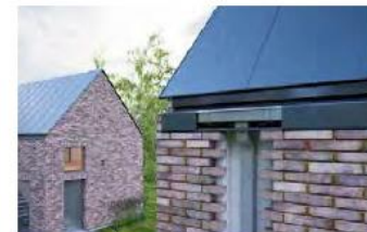
Zinc Roof with Hidden Gutters to Leading Edge and Central Valleys
