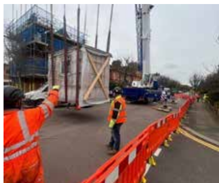
A crane lifting a bathroom pod
