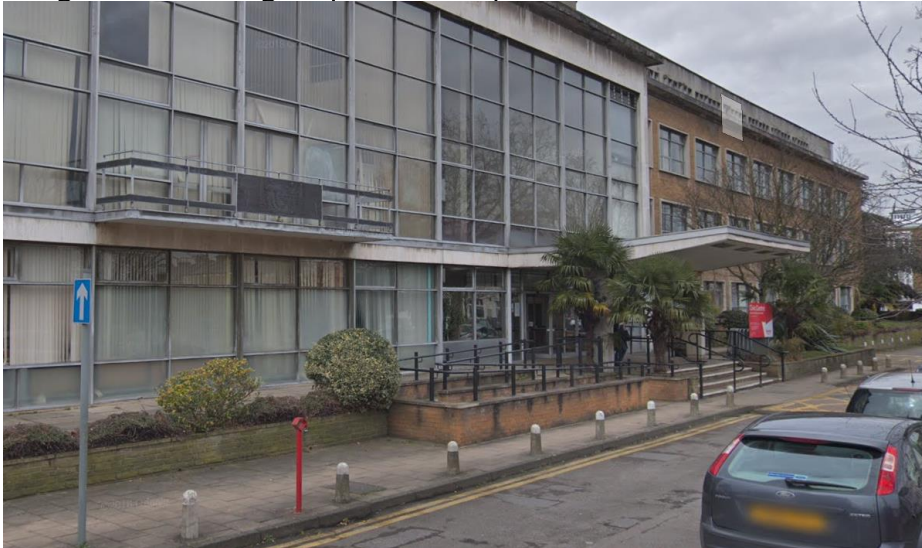
Image 11 - Existing steps and ramps to entrance
