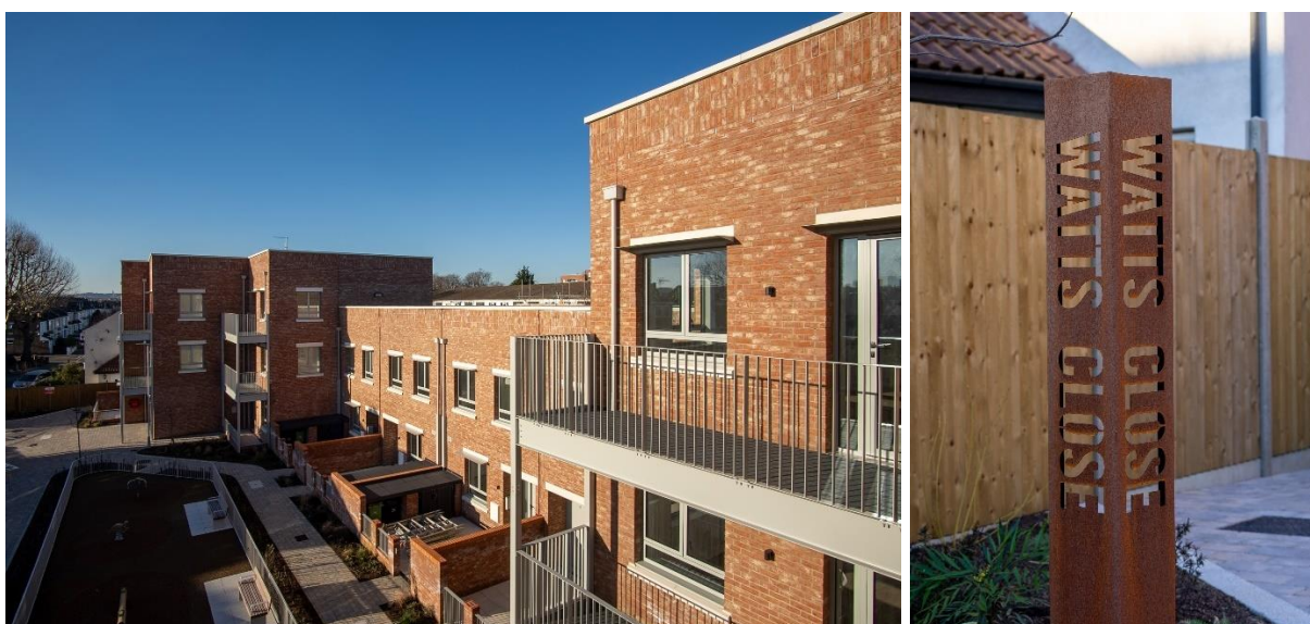
Figure 10: Aerial view of development with 16 new apartments accessed of Watts Close and two new houses accessed off Lomond Close. Photograph of the Watts Close signage.
