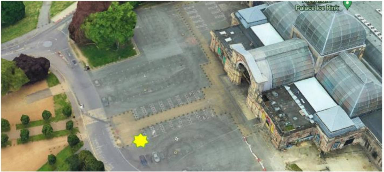
East car park – 3no pay terminals
