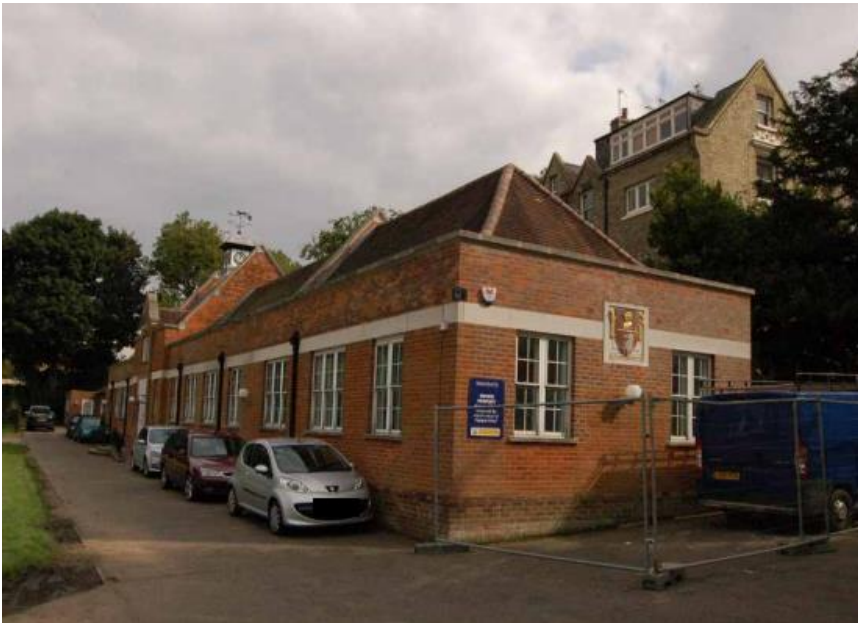
Figure 11: Existing Richards Music Centre
