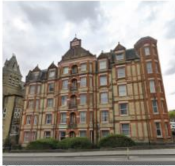
① Two tone brickwork and contrasting lintels
