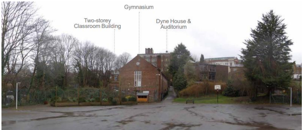
Photo of Rear Elevation
