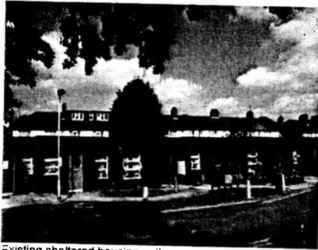
Existing sheltered housing units
