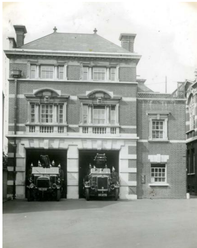
Photo 1: Fire Station operating within its intended use
